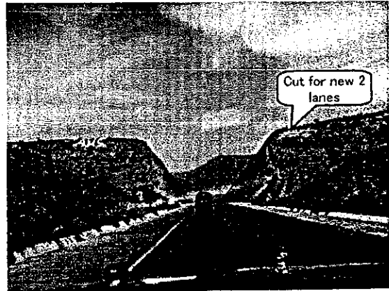
Direction (From Start Point to Tunnel) Estimated Quantity Common: 2,050 m 3 Rock: 38,900 m 3 Total: 40,950 m 3
