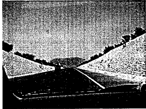
Direction (From Start Point to Tunnel) Estimated Quantity Common: 9,100 m 3 Rock: 3,900 m 3 Total: 13,000 m 3
