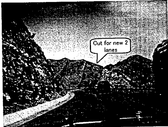
Direction (From Tunnel to End Point) No.N-2 : Sta.21.575 - Sta.21+725 (L=150m) Maximum Cut Height = 32m
