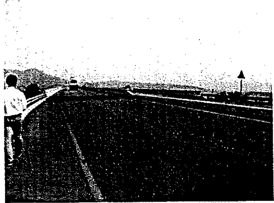
Direction (From Tunnel to N-80 Intersection)
